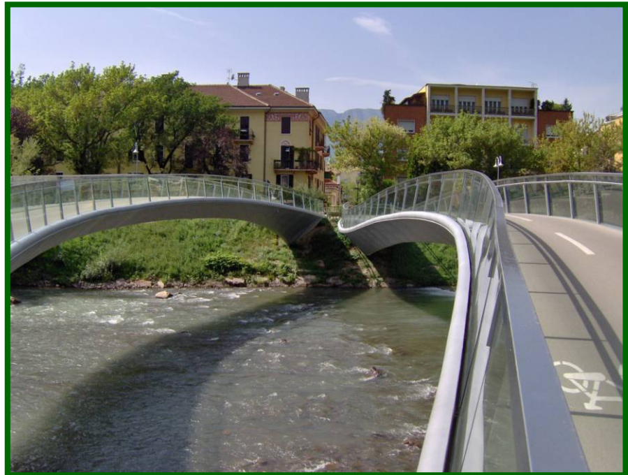
Cycle path on bridges
